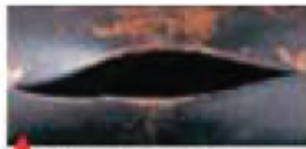
FREEZE RUPTURE Caused by low water flow in the evaporator.
